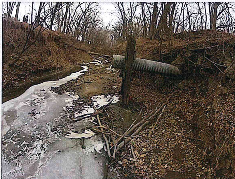
Photo 4. This 2011 photo shows an existing 18" CMP and pile bent structure exposed in the channel. The end of the CMP and pile bent structure were originally constructed at the edge of the channel bank. This photo shows how the channel has eroded approximately 10 feet wider behind the pile bent structure and 6 feet deeper than when originally installed.
