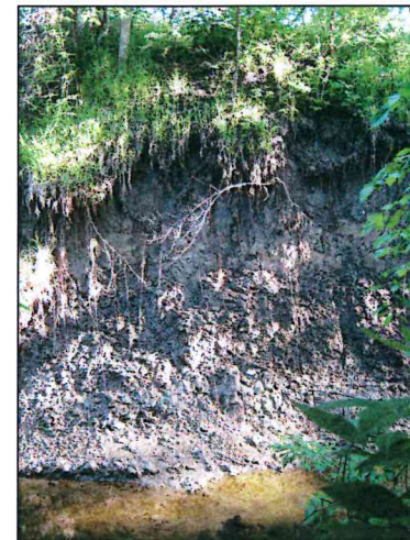
P8 - Creek Erosion
