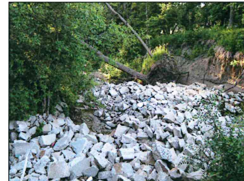
P10 - Creek Erosion
