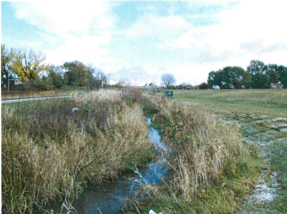
Current Channel along US 77 Looking North
