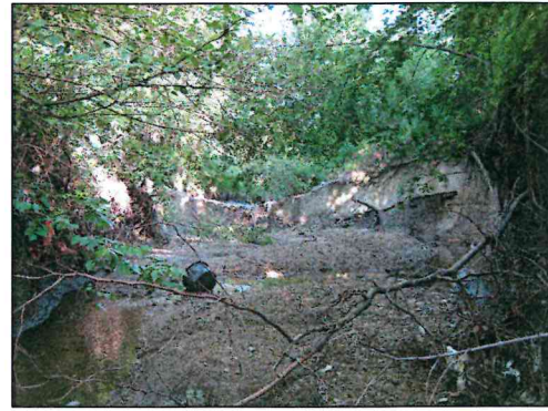
P5 - Creek Erosion
