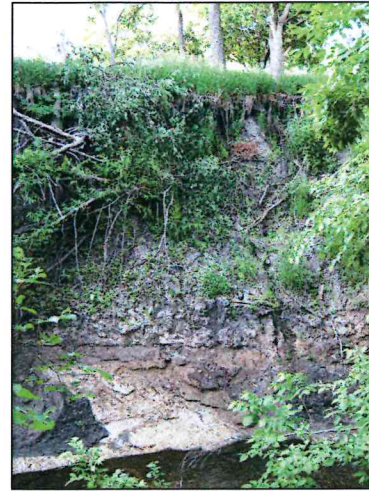
P6 - Creek Erosion
