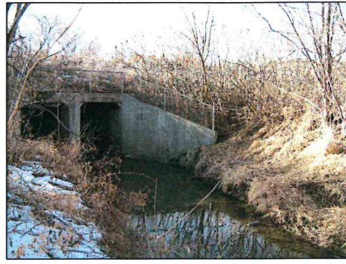
P1 - 160th Street Culvert
