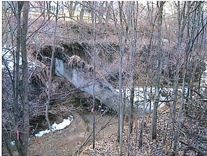
PHOTO 1: This 2011 photo shows the massive washout below the existing grade control structure and how water is being forced below the structure and along the bank. With further degradation, the vertical slopes may encroach on the sanitary outfall sewer located along the channel's south side.
