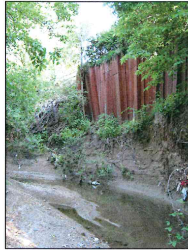
P3 - Steel Piling
