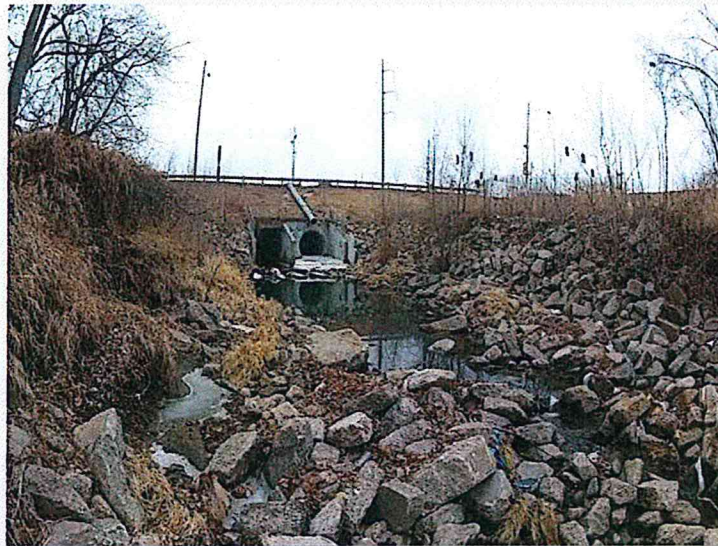
Photo 3. This 2011 photo is taken from standing at the outlet of the 8' x 10' box culvert and the 84" RCP culvert, while looking downstream. The significant washout and erosion along the side slopes can be seen. The large washout of rip rap and movement of rip rap downstream can also be seen in the photo.
